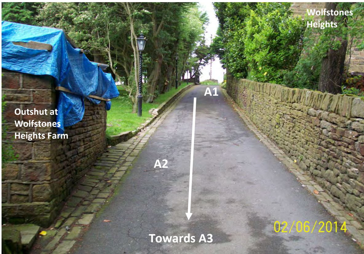
14. View west from near point A2 towards point A at Wolfstones Road. To the left (south) is an outshut forming part of Wolfstones Heights Farm. This part of the building had been damaged by fire in December 2013. 02 Jun 2014.
