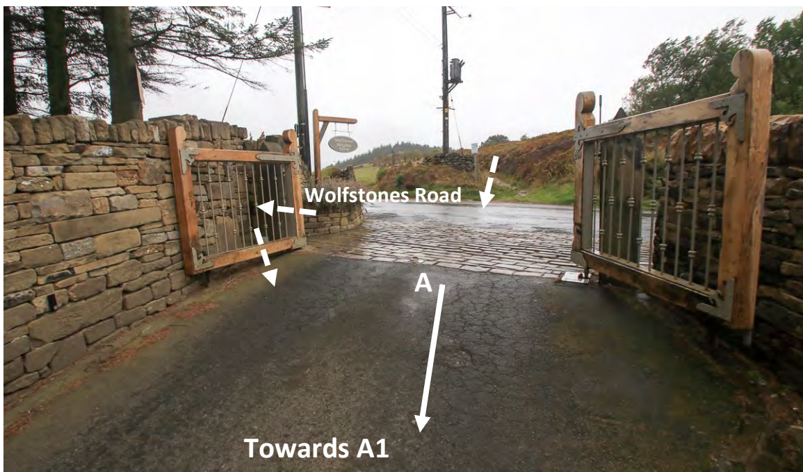
6. Electric gates at Point A and adjacent gap / stile. Looking west to Wolfstones Road. The wall to the south (left) was constructed in the period summer 2014 to summer 2017. Photograph supplied by the applicant. 08 Sep 2018.
