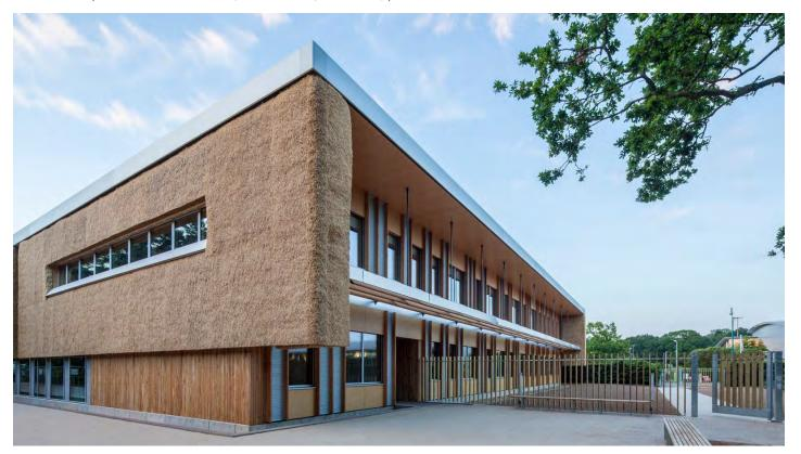
The Enterprise Centre at UEA has minimised the emissions associated with construction through the use of natural and recycled materials for every part of the building. This includes the use of:
