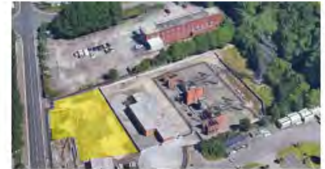
4. Northern Power Grid Substation
