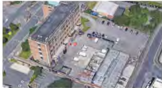
1. BT Openreach Exchange and Office
