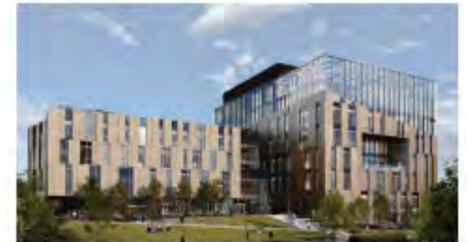
University of Huddersfield Health & Innovation Campus - Phase 1 building
