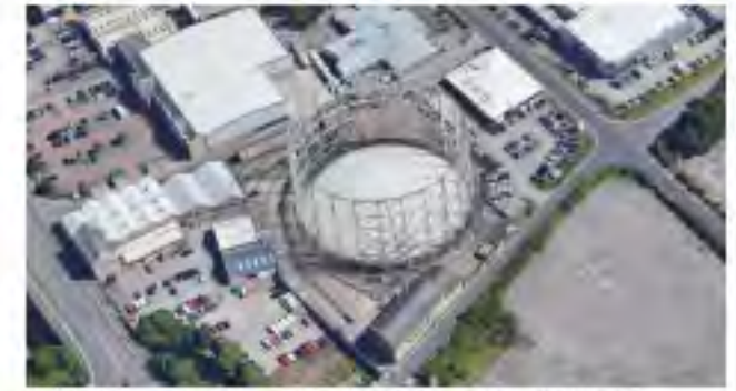
3. Northern Gas Networks Gasometer (gas holder)
