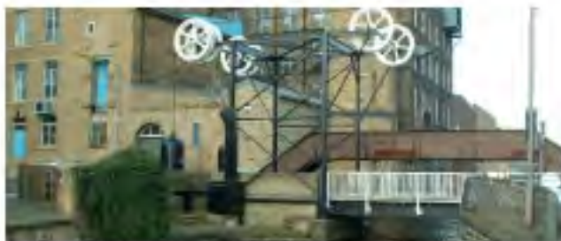
4. Locomotive Bridge and adjoining mill buildings
