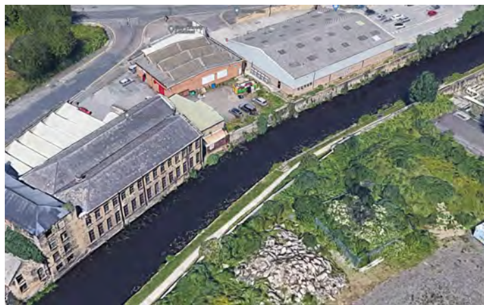
Aerial view of the existing conditions at the Canal and the lack of integration with its surroundings
