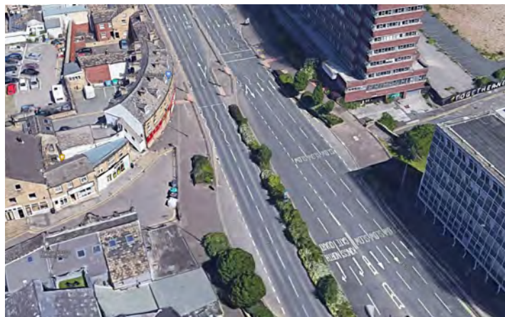
Aerial view of the existing A62 Ring road and pedestrian junctions
