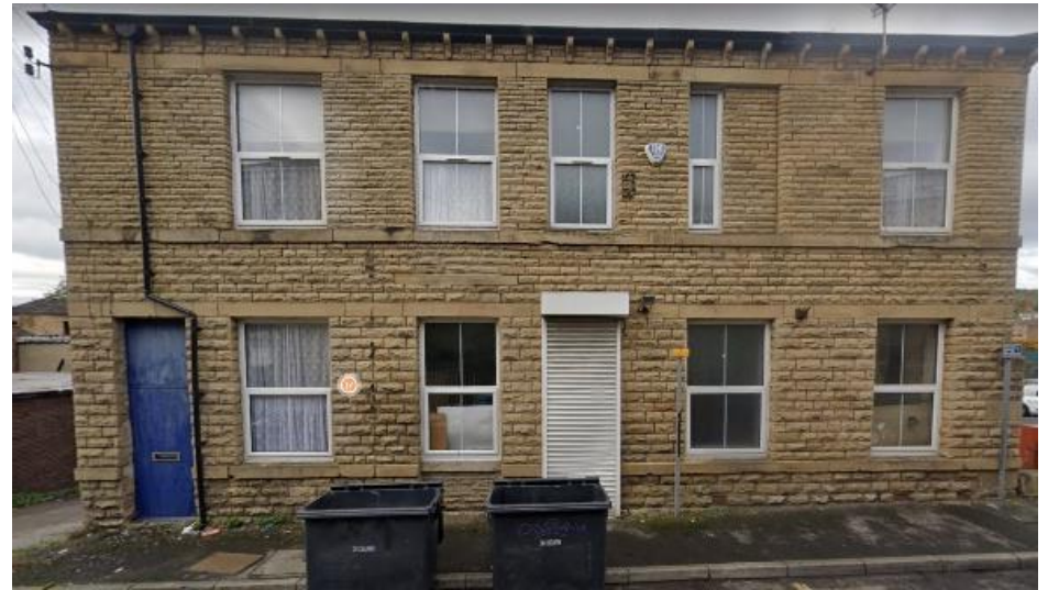
Edward Latham House
