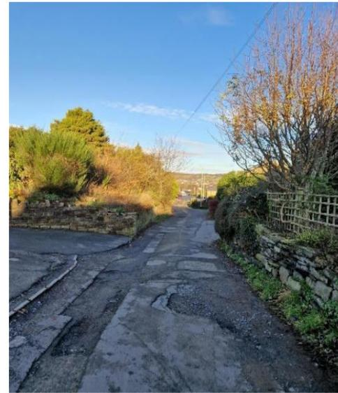
*Photo 8: Privately maintained section of Colders Lane for private carriage access to residential properties. Uneven surface with several layers of tarmac.*
