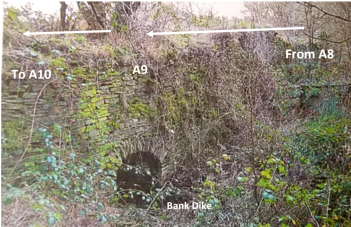
29. Culvert carrying Bank Dike beneath Meltham 70 at point A9. This 'bridge' is referred to in various User Evidence Forms. Photo supplied by Applicant 1 in Jan 2016.
