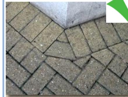
Paving laying should be orientated to follow the grain when using paving chamber covers.
