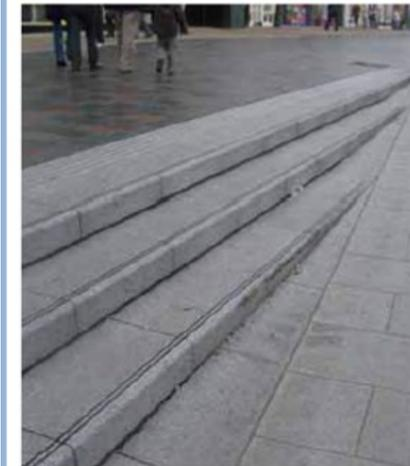
Access ramps should be an integral part of the scheme and should be made into a feature where possible.
