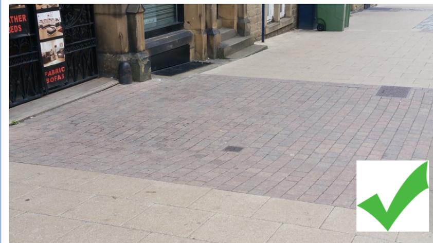
Vehicle dropped crossing details to be made up in small Tegula sett details which allow them to follow the contours of the ground better. This gives a better result
