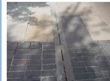
Drainage should be carefully considered, slot drains are aesthetically pleasing within a scheme, but the width of the gap should be considered to avoid trapping debris and cigarette butts, which inhibit the drains function.
