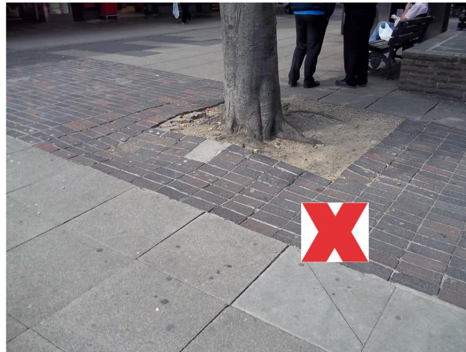
Rigid paving construction ensures the longevity and durability of the finished surface, unlike flexible paving systems which sink, move and distort. Street reinstatement works should be carried out in accordance with: [https://www.gov.uk/government/uploads/system/uploads/attachment\\_data/file/4382/practicalguidetostreetworks.pdf](https://www.gov.uk/government/uploads/system/uploads/attachment_data/file/4382/practicalguidetostreetworks.pdf)
