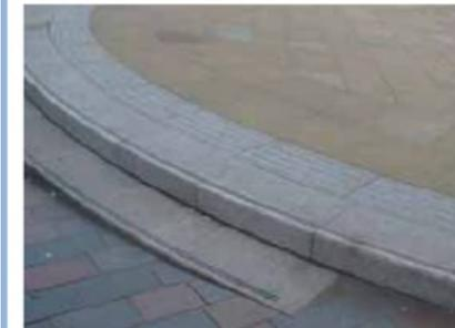
The image left shows good use of paving in a pedestrian crossing. Depending on the location and whether gold, silver or bronze standard is required, the tactile paving could be insensitive and a more subtle attractive use of natural stone tactiles or crossed brass studs as seen below would have been more appropriate.
